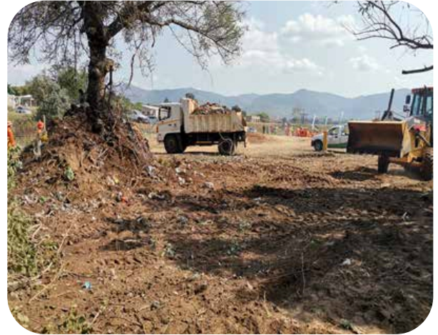
Grader and trucks clearing debris
